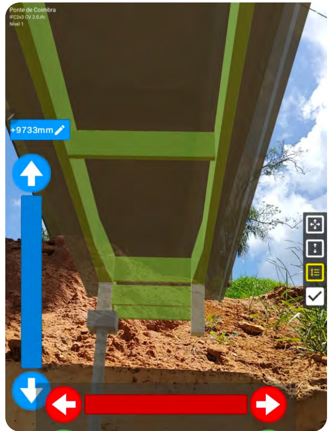
Adjusting the x, y, and z coordinates of the BIM model overlay on the bridge in GAMMA AR during on-site inspection.
