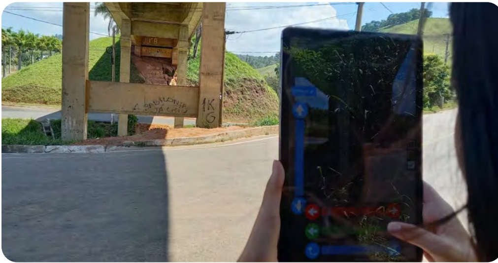
Using GAMMA AR to overlay the BIM model onto the Coimbra I Viaduct for structural inspection. 1
